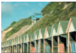
Along the promenade The beach huts along the length of the promenade at Bournemouth are owned by local people who use them year round. A passenger lift provides access up and down the steep cliff face
